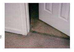
undercut below the door into the hall or main part of the house. Dirt/dust particles in the bedroom air are impacted onto the carpet underneath the door. Over time, enough particles build up, causing a dark stripe on the carpet at the threshold.
