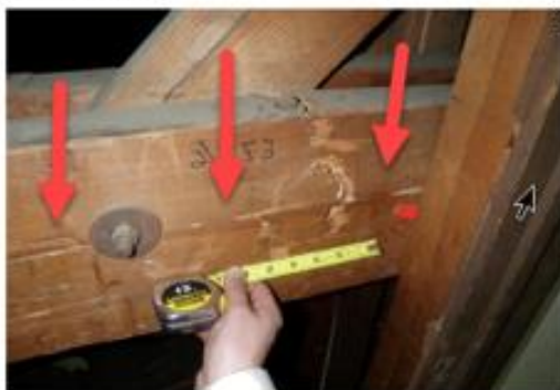
Figure 9: Termite infestation in bottom chord of a powder post beam
