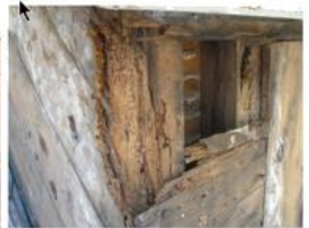
Figure 5 Termite damaged timber
