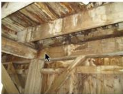
Figure 3 Discoloration can be a sign of rot
