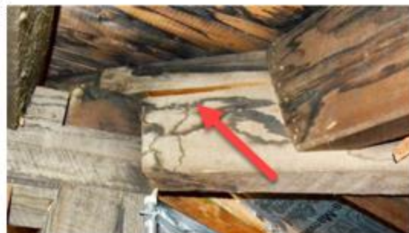
Figure 10 Split in a notched timber
