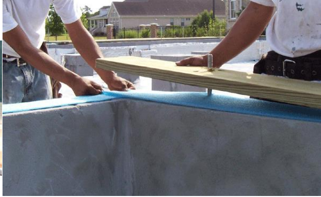
Simple sill seal (capillary break)
