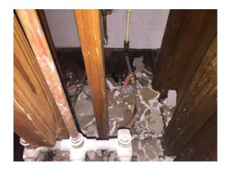
I'd used that shower a few times over the years and always wondered why the pressure was so low. Now I understand. The plumbers installed the valves but then didn't open them fully. Those red handles should be straight in line with the pipes. Nice!
