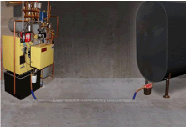
Surface view of a properly protected (sleeved) buried copper fuel line
