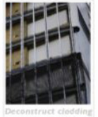
Deconstruct cladding (Q3 2023-Q2 2024) & structure (Q1-Q4 2024.)
