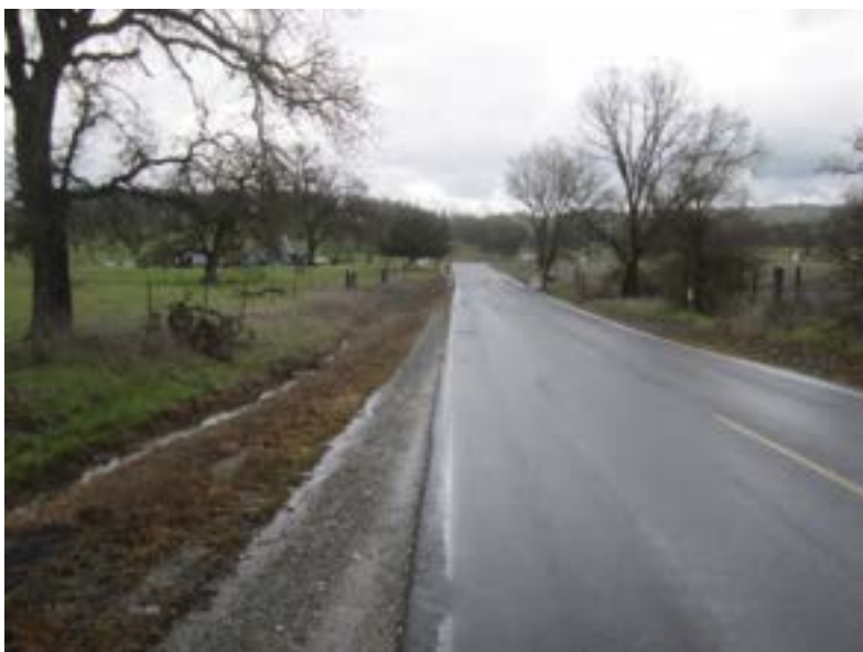
Figure 22. Key View 3—Existing Condition Facing Eastbound
