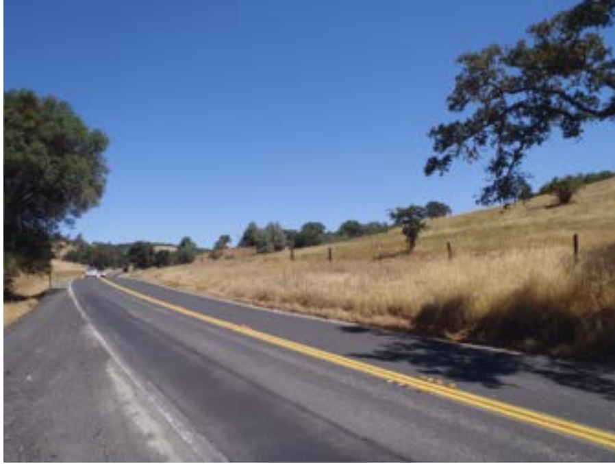
Figure 16. Key View 1B-Existing Condition Facing Eastbound
