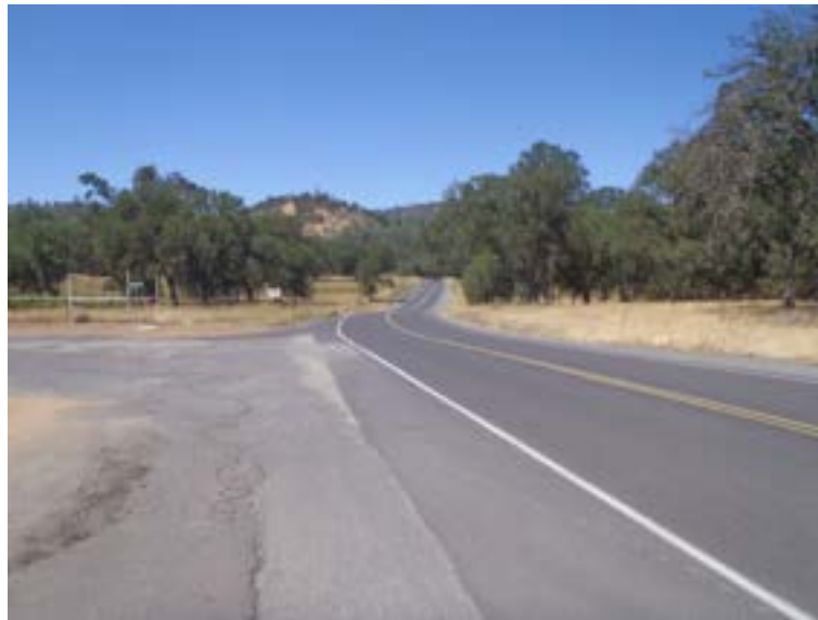
Figure 18. Key View 2—Existing Condition Facing Westbound
