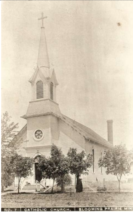
The old church, 1877-1928 (Built by Fr. Pribyl of Owatonna)
