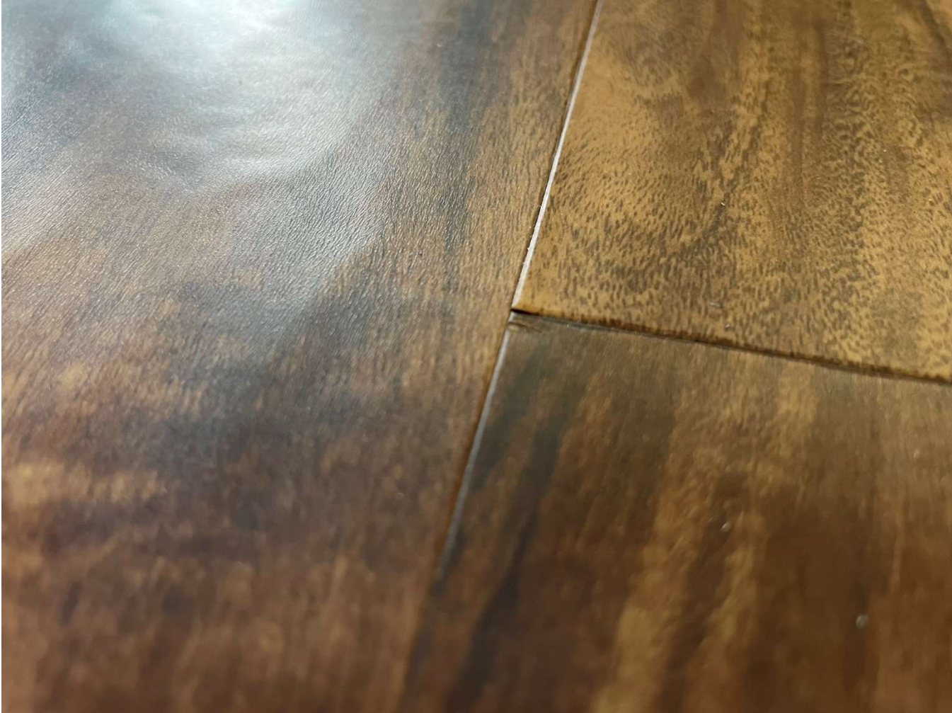
Damaged corner
