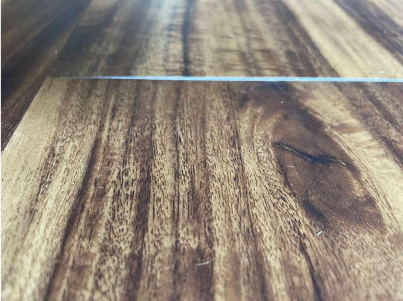
Disengaged end joint
