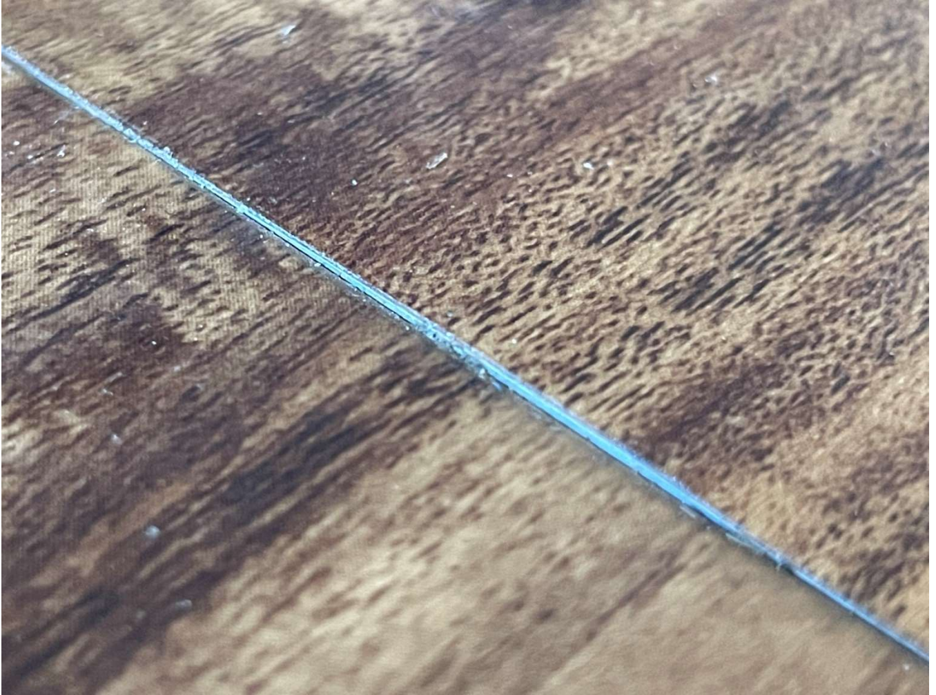
Close up of disengaged end joint
