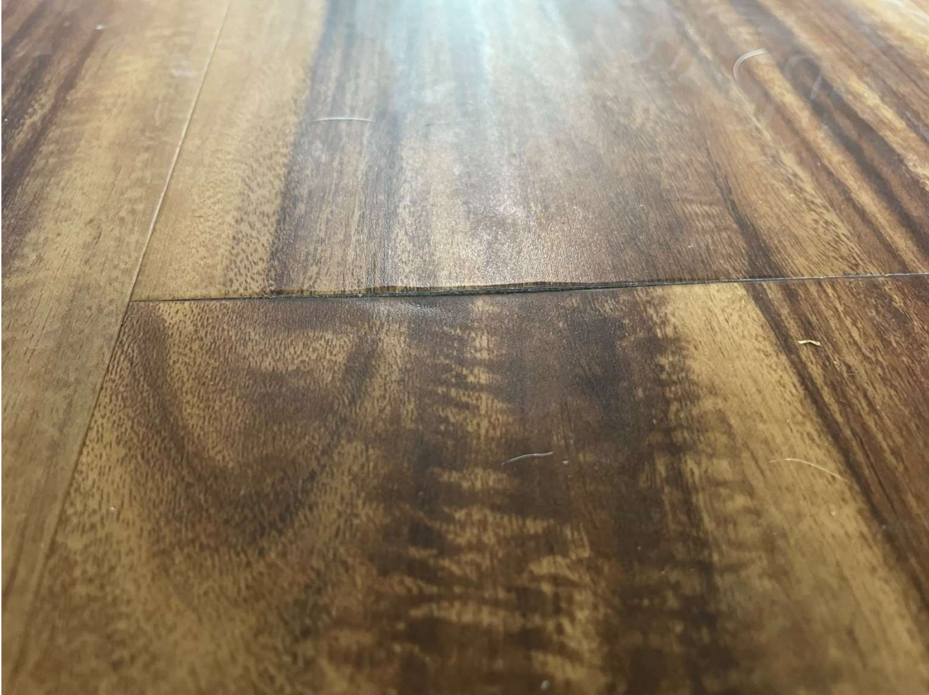
Disengaged end joint- deflection
