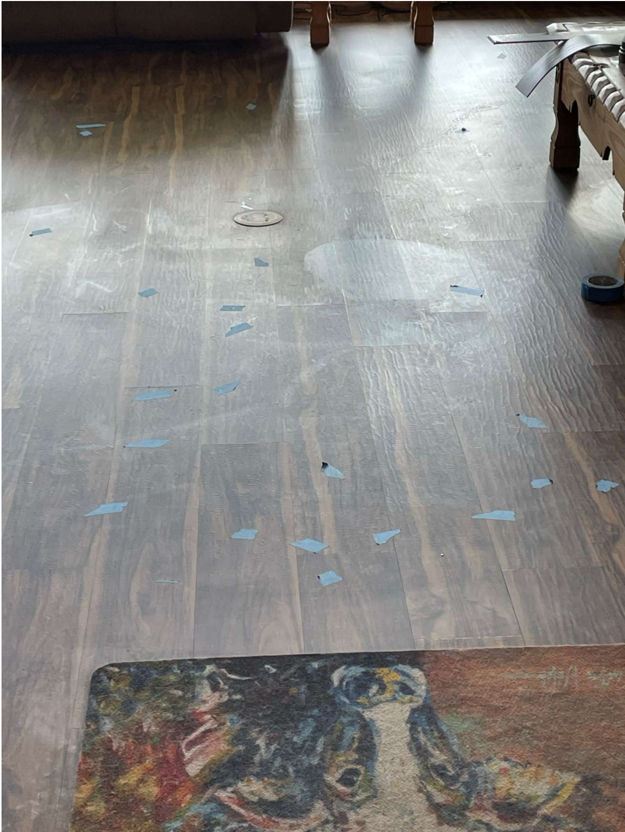
Haze on product after cleaning, Small spot shows test cleaning by customer.
