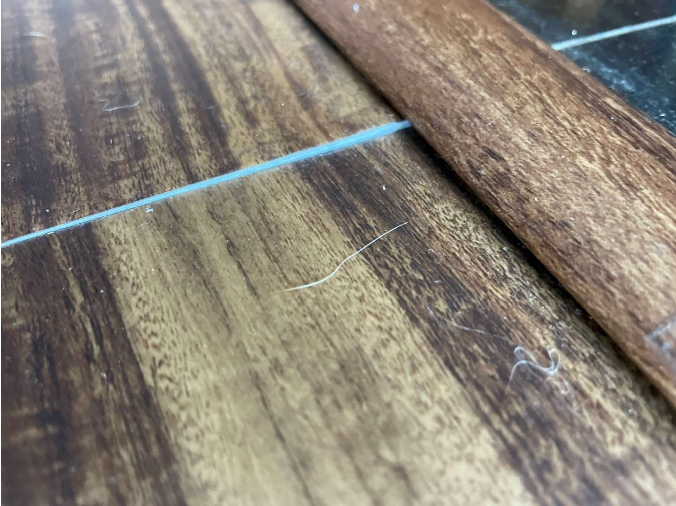
Disengaged end joint
