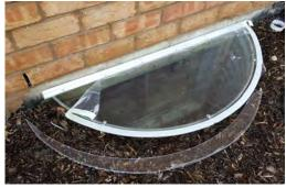
note: when masking the profile of the well we recommend keeping the tape to the outside of the well creating an overhang much like the drip edge on a roof. This will allow the water to drip outside the well
