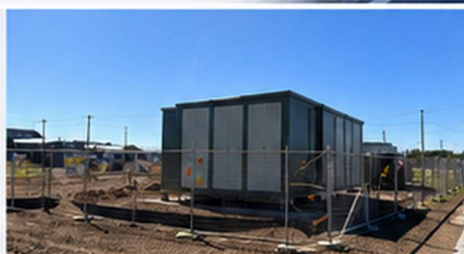
Yarrabilba – P4 under construction
