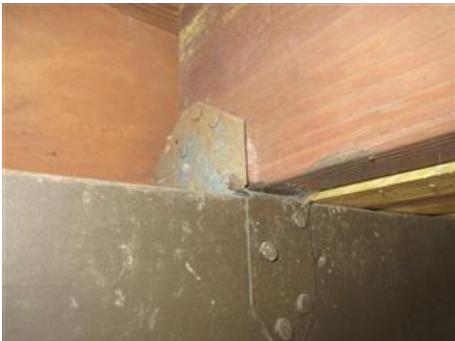
Roof to Wall 1
