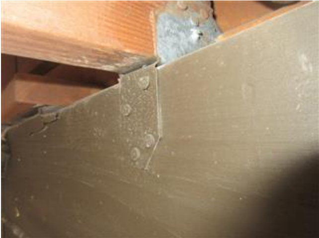
Roof to Wall 2
