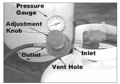
Photo 6: Adjustable pressure regulator assembly
