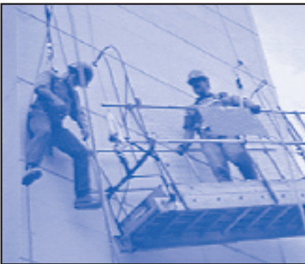
On single-point and two-point adjustable suspension scaffolds, workers must be protected with guardrails and personal fall-arrest systems.
