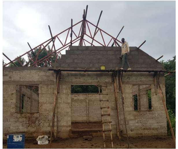
Trusses and purlins in place and gables going up on church in Marangu. We plan to dedicate the new church on our August trip.
