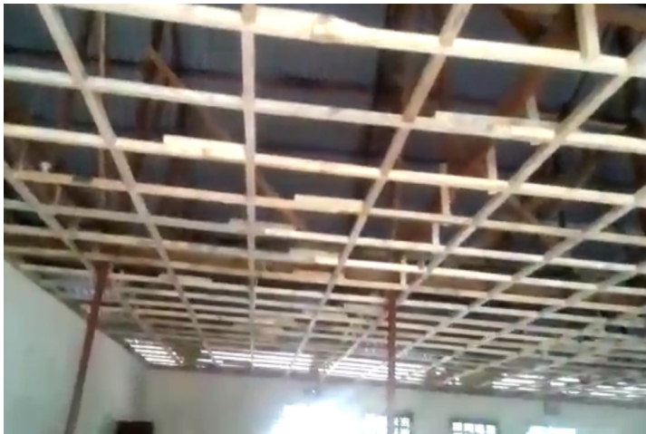
New grid for installing ceiling panels in the dining hall
