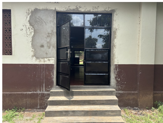
A new door in the cafeteria. This allows access to the dining hall from both sides of the building.
