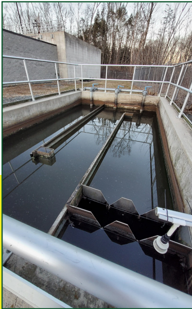
The tank after cleaning, this is how cleanliness should look.
