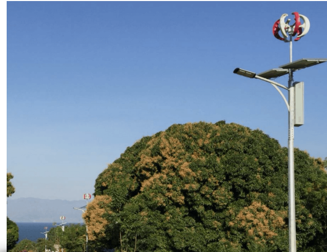
Supplying Street Light & Water Project
