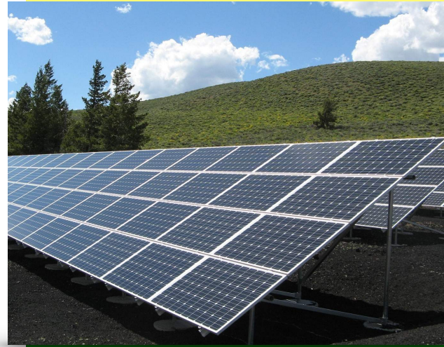
Solar Power Plant Project
