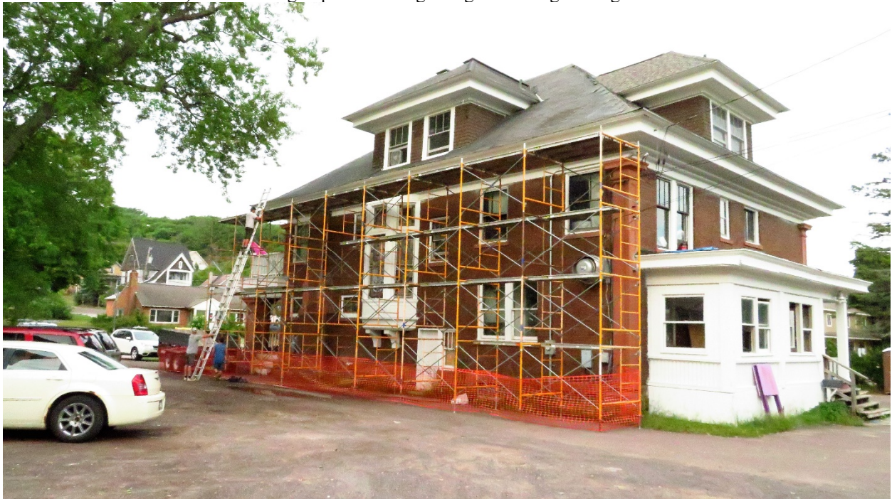
Side of house (East face) – scaffolding in place and beginning of existing roofing tear-off.
