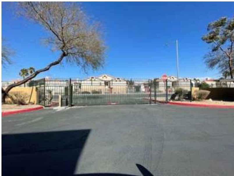
The Entrance Area Category Components include the Gate Replacement, In Ground Loops, Loop Detectors, Motors, Pedestrian Gates and the Key Pad Entry System. The Gate Components Estimated Remaining Useful Life are an estimation only.
