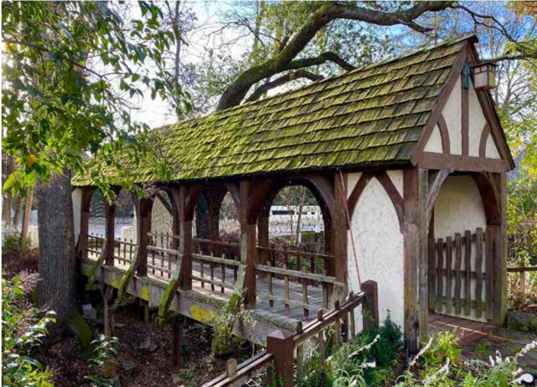
The “Donna Linda” Bridge 2145 Alameda Diablo Architect: Will G. Corlett Architectural Style: Arts and Crafts Built in 1928
