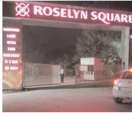
ROSELYN SQUARE project construction site.
