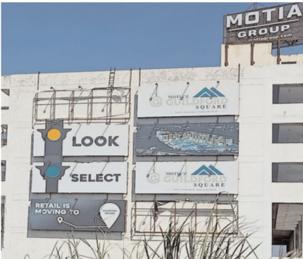
MOTIA GROUP project construction site.
