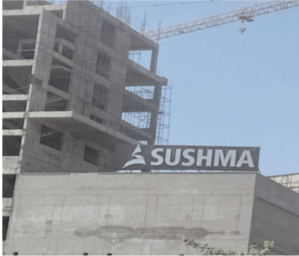
SUSHMA project construction site.
