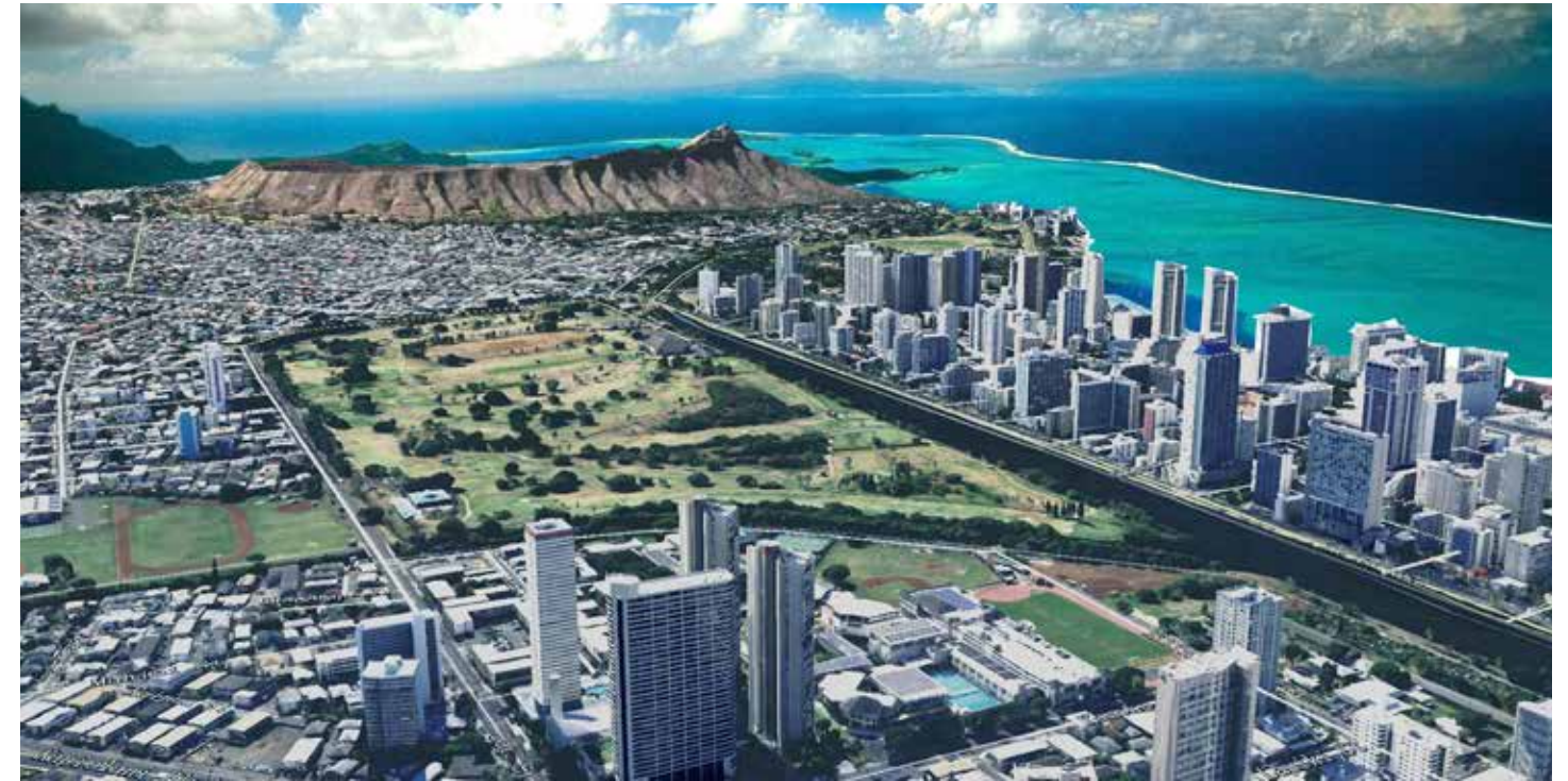
Original image of golf course. Shows disconnected Waikiki, minimal water flow that impacts the water quality and how this is a flooding hotspot.
