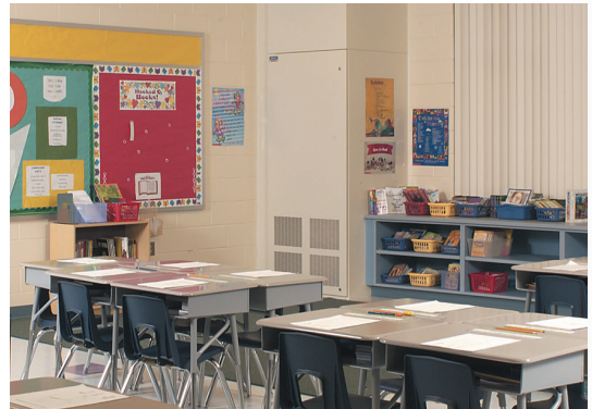
School service technicians need to only open the doors of their Airedale Classroom HVAC units to have easy access to the controls.
