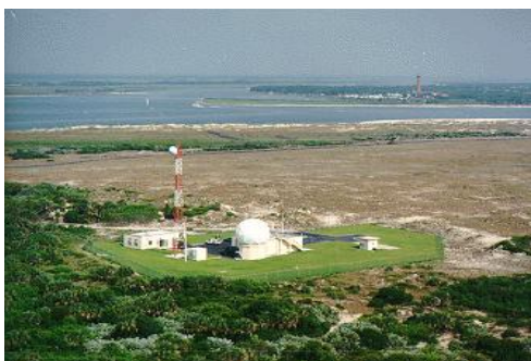
Ponce De Leon (PDL) Tracking Station
