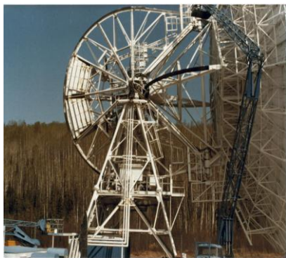
26M Counterweight Replacement
