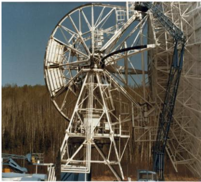
26M Counterweight Replacement
