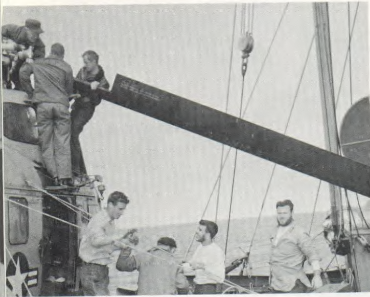
VX-6 CREW PUTS ROTOR BLADES ON WINDMILL
