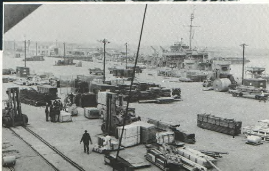
DOWN THE HATCH goes a Caterpillar tractor as the WYANDOT receives cargo from crowded dockside. Jumbo fork lift trucks brought supplies to ships, 30-ton ship's cranes swung cargo on board and down into waiting storage areas in hold.
