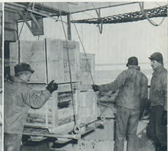
Work-rushed Seabee, right, starts pre-heating unit to warm up tractors hauling unloaded cargo from bay ice inland.
