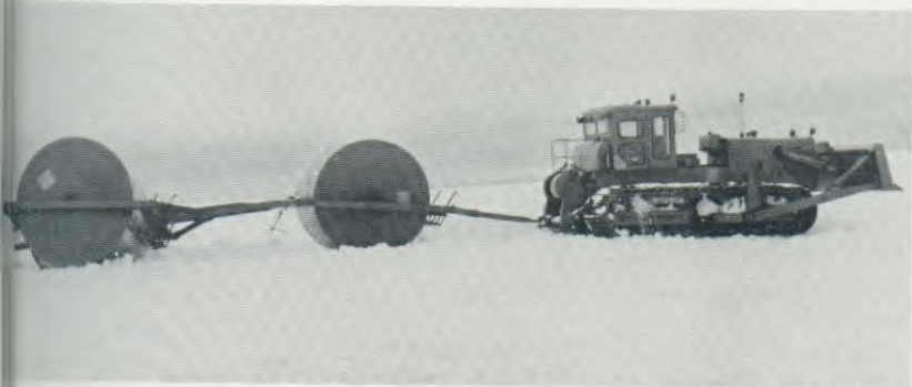
TRACTOR weighing more than 35 tons draws two 30-ton rollers as it levels snow for the Kainan Bay area for site of Little America. Right, William Bureson, CM2, adjusts oil filter on D-8 tractor.
