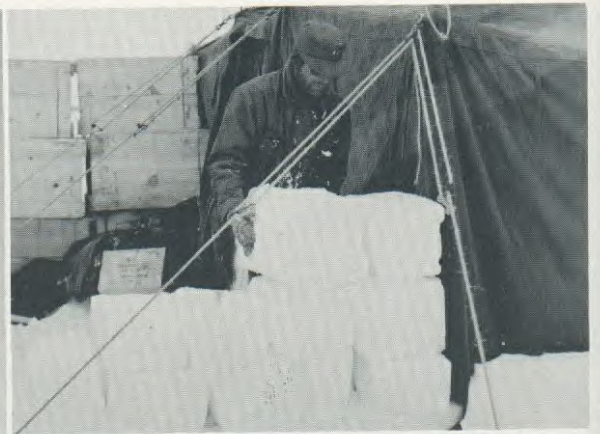
SNOW-BLOCK WINDBREAK AT GALLEY
