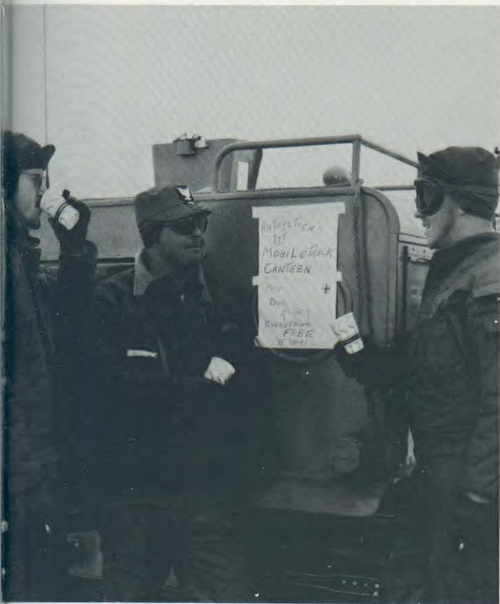
COFFEE BREAK during construction at Little America. "Doc" Koller, HM2, center, plays mine host to Seabees.
