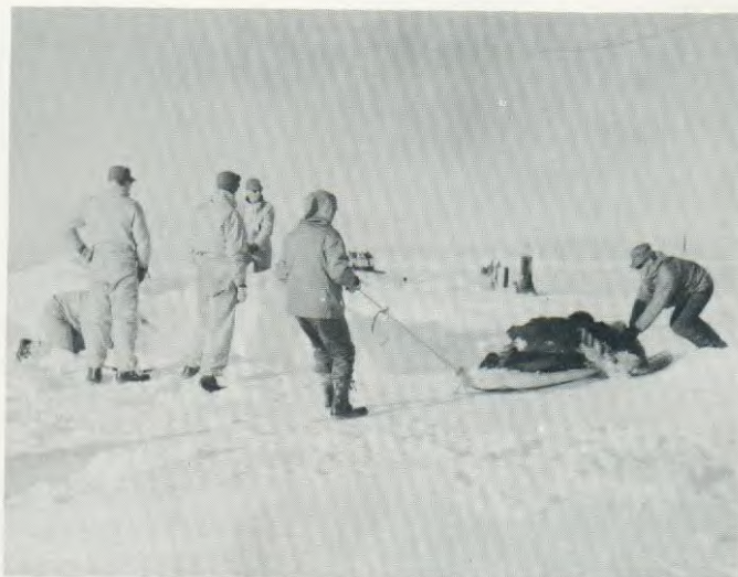
DEADMAN, log with metal harness and ship's lines attached, is placed in hole dug into shelf ice far inland.
