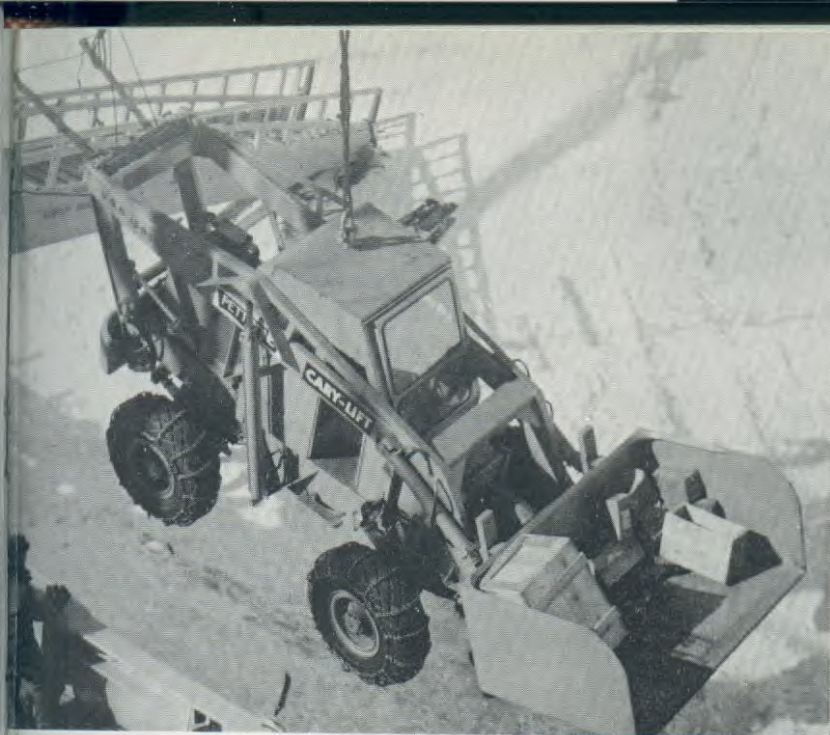
CARY-LIFT WITH DUNNAGE IS SET DOWN ON SHELF ICE
