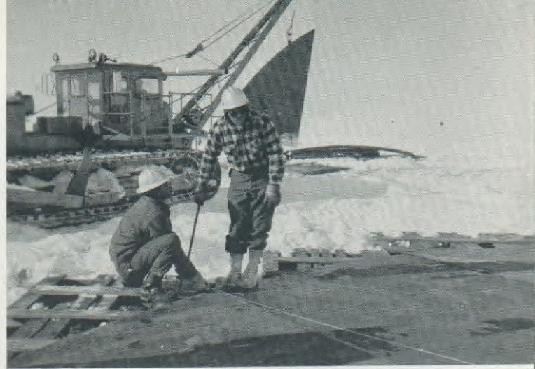
SQUARING UP PLATE AS LAST ONE APPROACHES
