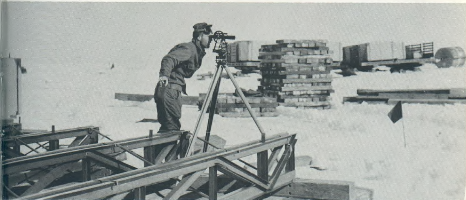
SURVEYOR CHECKS READING DURING LAYING OF FOUNDATIONS FOR BUILDINGS OF LITTLE AMERICA
