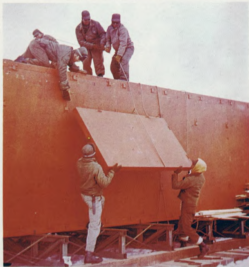
SEABEES hoist roof panel of Clement hut into place at LA-V. These prefabricated huts will house men of wintering-over group.
