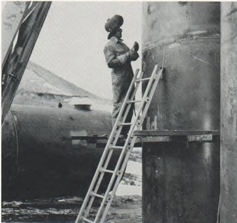
This 74-foot diameter by 8-foot high fuel oil tank was erected at McMurdo Sound, Antarctica, for the United States Navy.—Official United States Navy Photograph.
