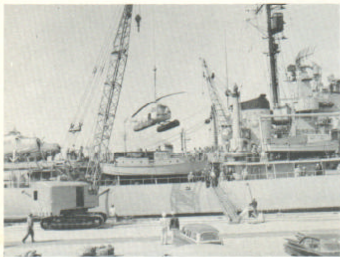
Loaded . . . make preparations for getting underway
