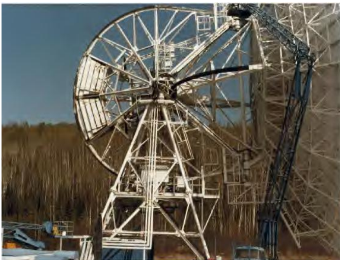
26M Counter Weight Replacement
