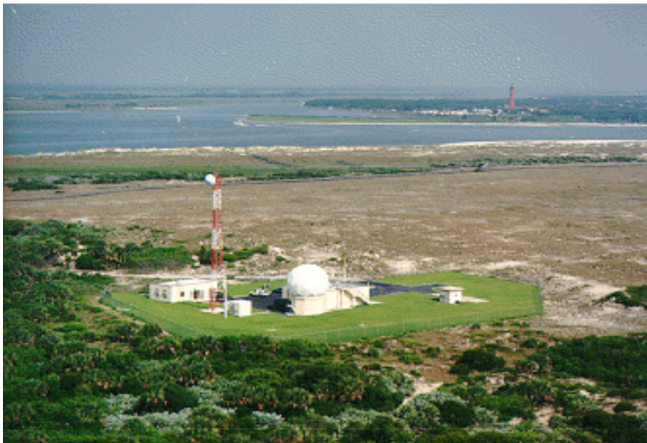
Ponce De Leon (PDL) Tracking Station
