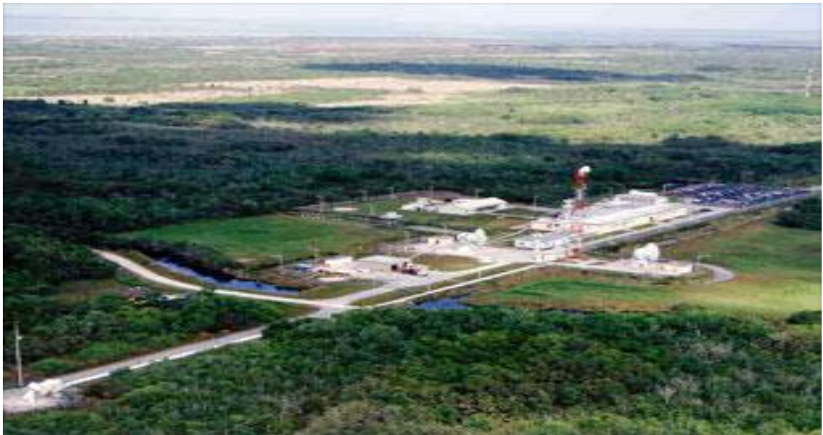
Aerial view of the Merritt Island Launch Annex (MILA). (NASA)
