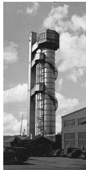
Buoyancy Ascent Tower
