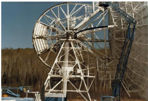
26M Counterweight Replacement
