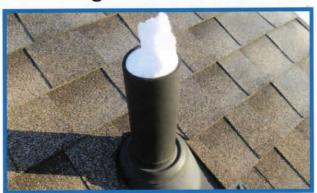
**OUR KIT** is a patent pending product. It works by bringing heat up from lower down in your plumbing stack, to the top not allowing frost to form.
