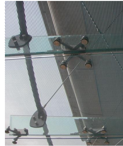
BOW TRUSS WITH TENDON & GLASS BEAM HYBRID CANOPY – BMW SHOWROOM. BANGALORE
