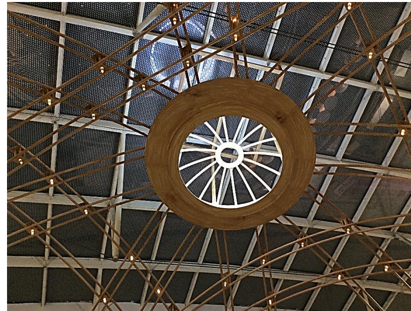
9M DIA. ALMN. TRUSS DOME. SUSPENDED FROM CEILING WITH TENDONS. CUSTOM MADE LIGHTING INSTALLATION
