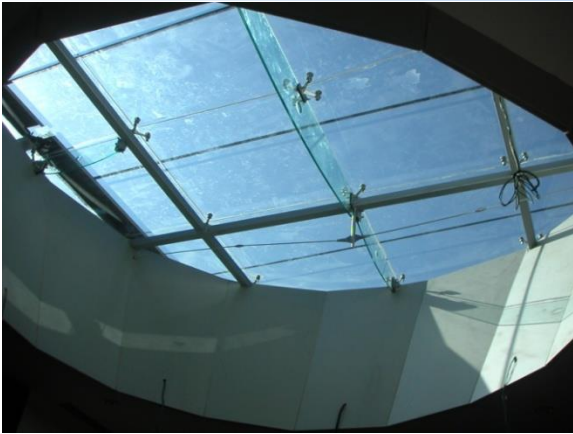
SS TENDON & GLASS BEAM HYBRID SKY LIGHT – INSILICA. BANGALORE
