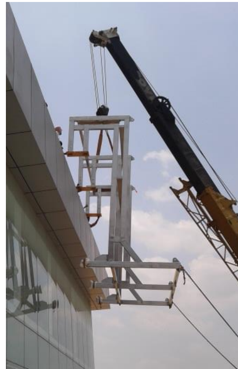
ON-SITE INSTALLATION with BOOM CRANE
