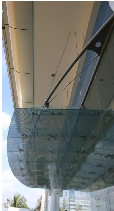
SS TENDON & GLASS BEAM HYBRID SKY LIGHT – INSILICA. BANGALORE
