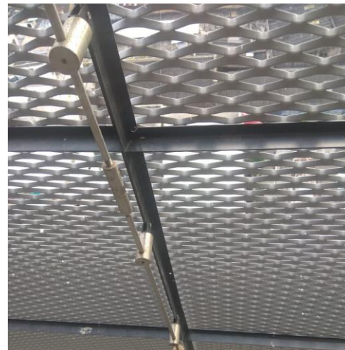
BESPOKE SS TENDON TRUSS
