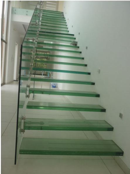
(8CT+2SGP+12CT+12CT)mm; surface #1 ANTI-SKID ACID ETCHED
