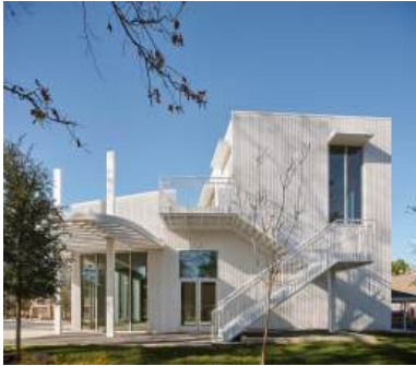
Self-Cooling Concrete: Modu x Transsolar concrete is cast in a corrugated pattern that dissipates heat.
