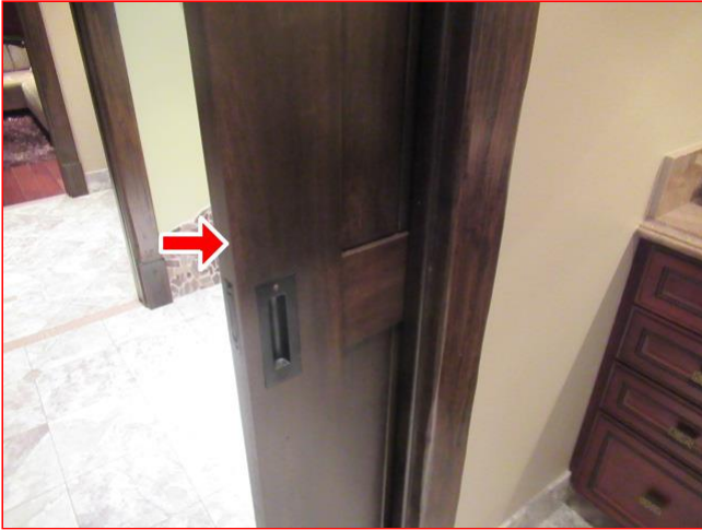
8.1 Item 1(Picture) (2) Some guest bedrooms doors do not latch.
