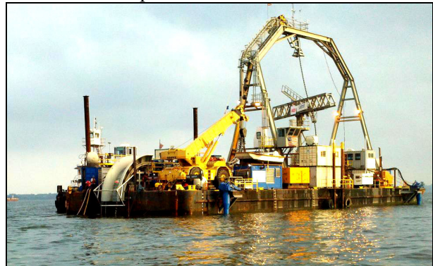
Figure 8: Submarine cable laying barge
