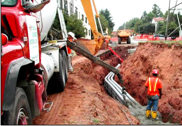
Figure 6: Open-cut trenching for duct bank installation
