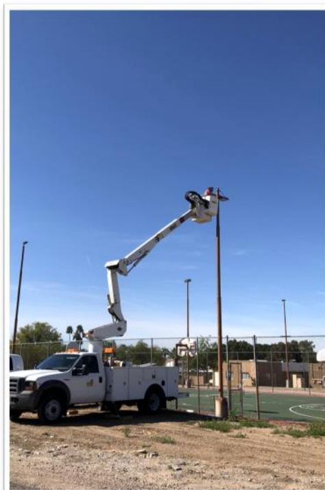
Repairing the lighting for the basketball court..
