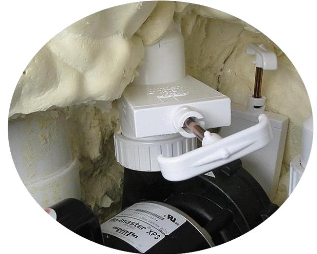
A small dripping leak out of a fitting in the equipment compartment can account for a 2" - 12" a day leak.
