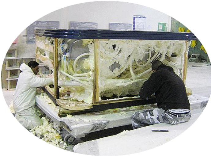
If you are still unable to find the leak and have confirmed that a leak exists and have excluded the potential of an equipment leak, all the foam will have to be removed to completely expose the plumbing, after which the leak will be visibly exposed.
