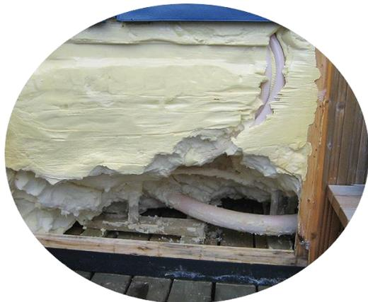
Once the area is exposed the spa must be filled so that the drip or leak can be visually confirmed.
