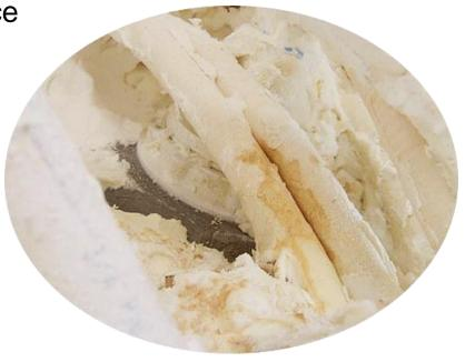
Make sure the area is clean and smooth before installing a new component. After installing and tightening a new jet body or other component, apply a generous layer of silicone sealant around the gasket perimeter and fiberglass under the shell as an added measure of future leak protection.
