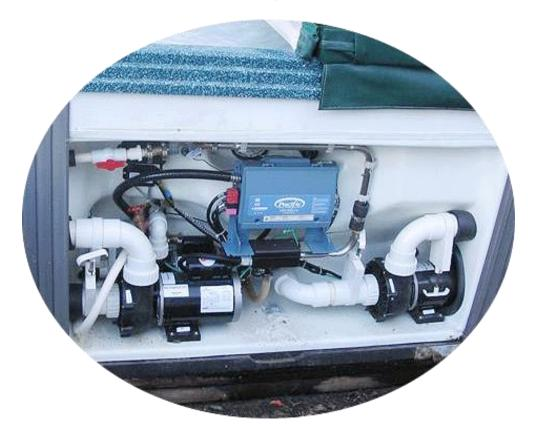
A loose fitting can be tightened. A small seepage can be siliconed. But a cracked pump housing or a split or corroded heater will require a component replacement.
