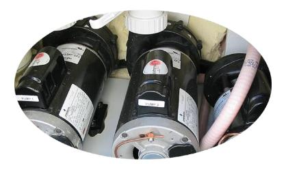
A small dripping leak out of a fitting in the equipment compartment can account for a 2" - 12" a day leak.
