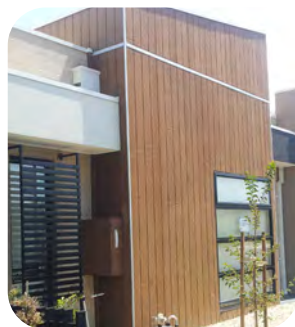
4 MONTHS: The board shows signs of lightening.
