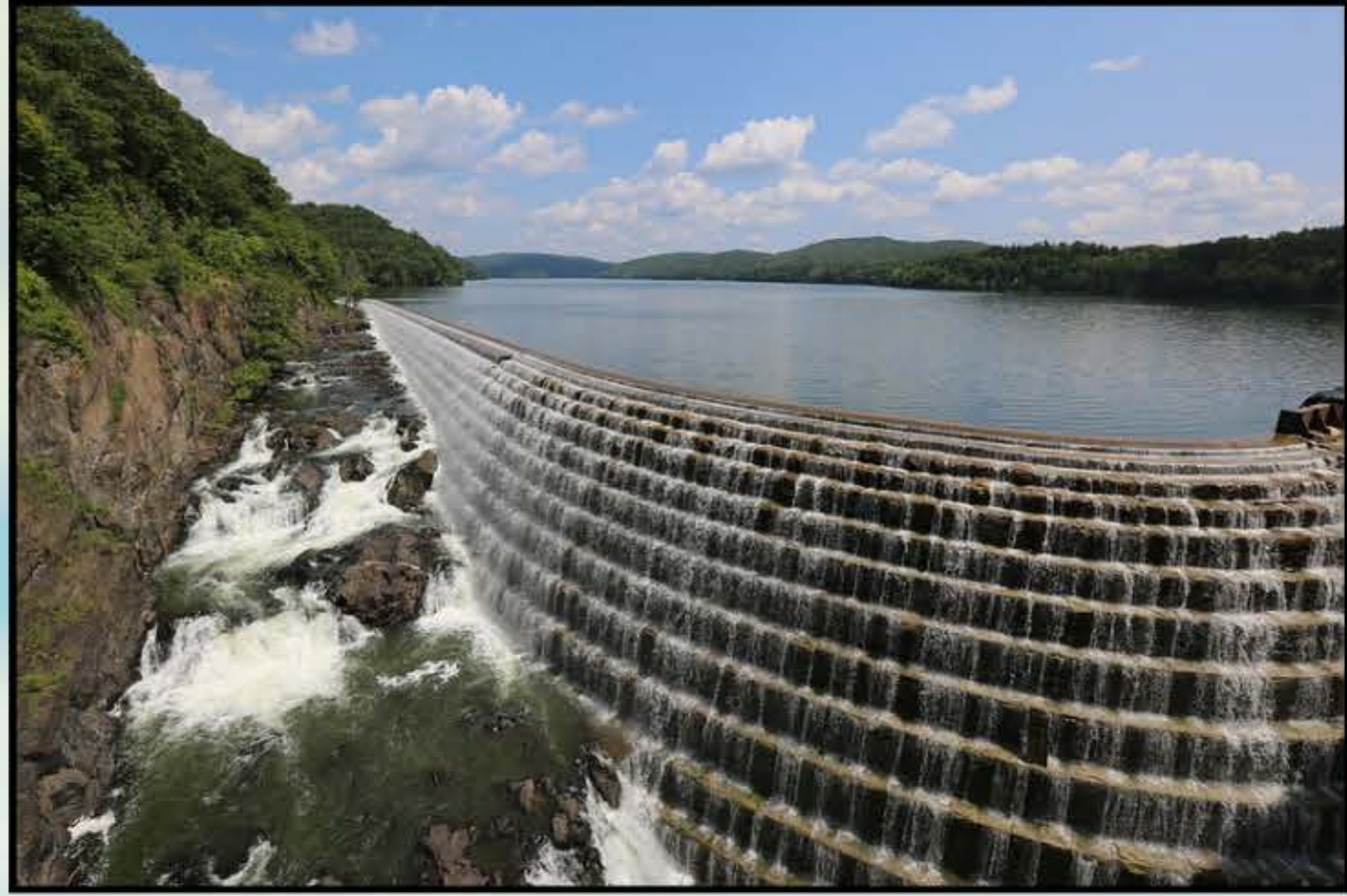
New Croton Dam Spillway - NYC Water (2025)
