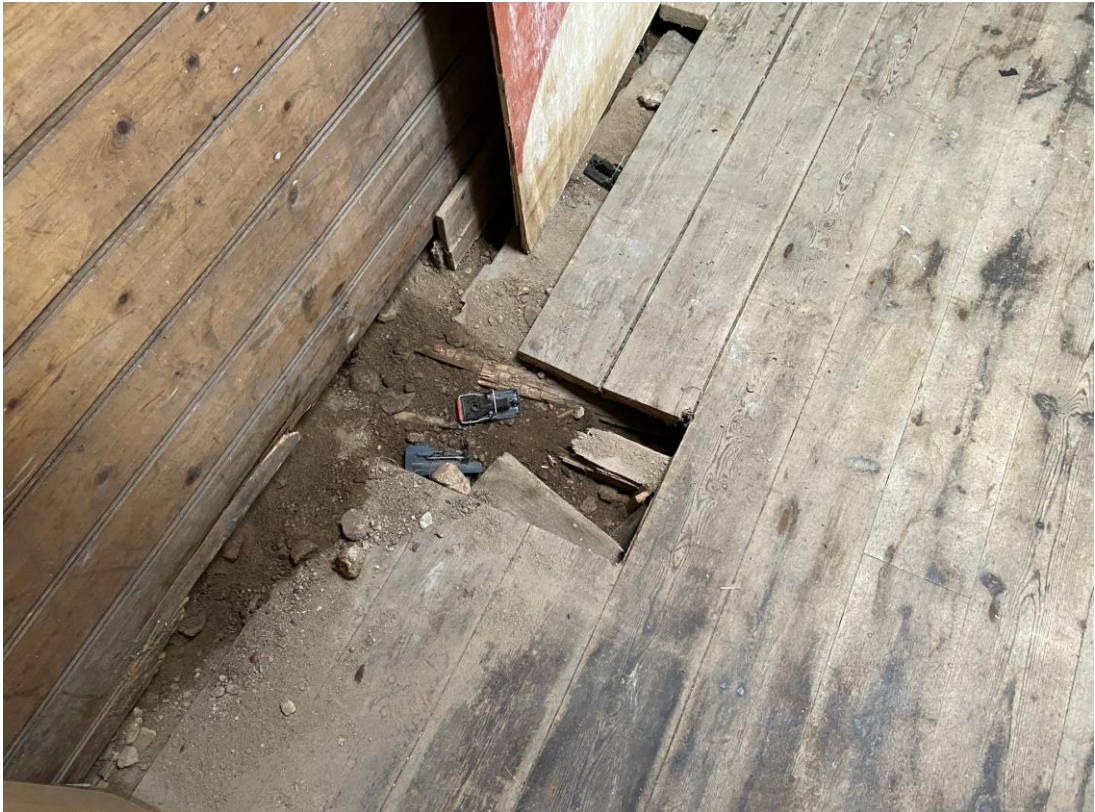
Photo 7: Rotted Floor, West 'Lean-to' Section
