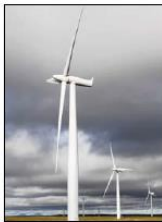
Strathly North has 23 turbines and started operating in 2015.
