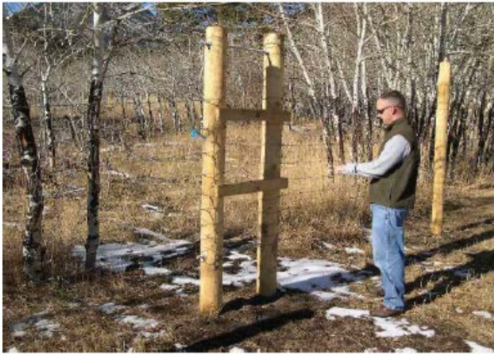
Figure 14: Ladder/stile crossing structure Photo by Kurt C. VerCautern, USDA
