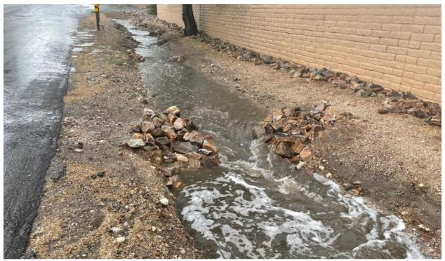
*Figure 6. An example of a series of one-rock dams along a neighborhood street to reduce erosion and enhance infiltration.*
