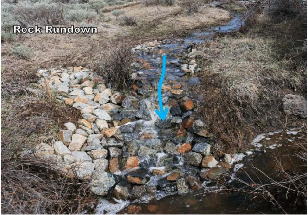
Figure 7. An example of a hand-placed rock rundown to control stormwater down a slope and into a channel.
