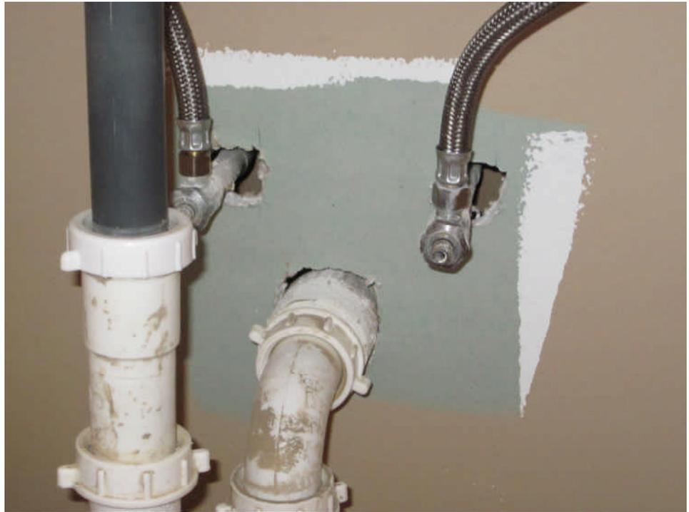
There are no shutoffs installed for both hot and cold water pipes under the basin.
