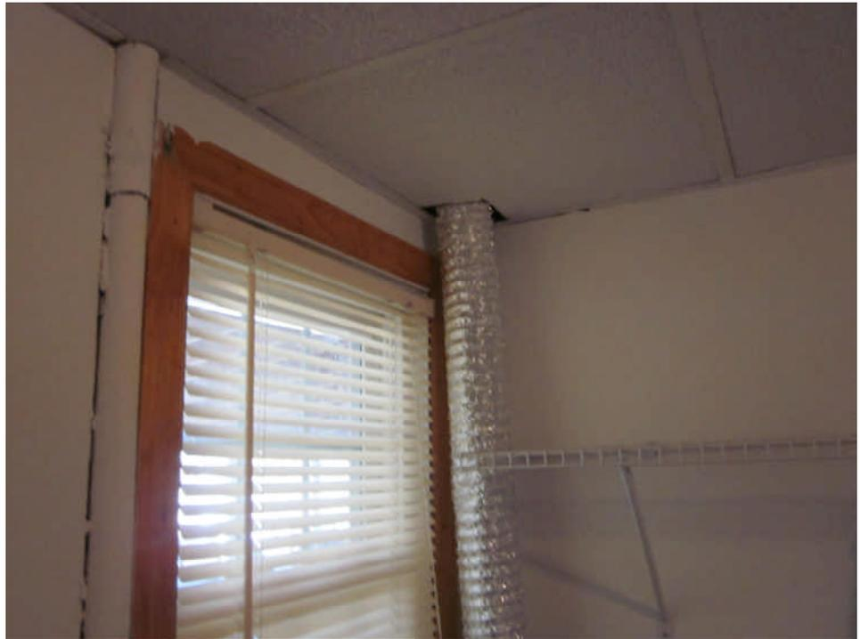
The windows are very tight and tough to open; further investigation is needed to determine the cause of this. Is it possible that the wood frames have swelled due to flooding issues?
