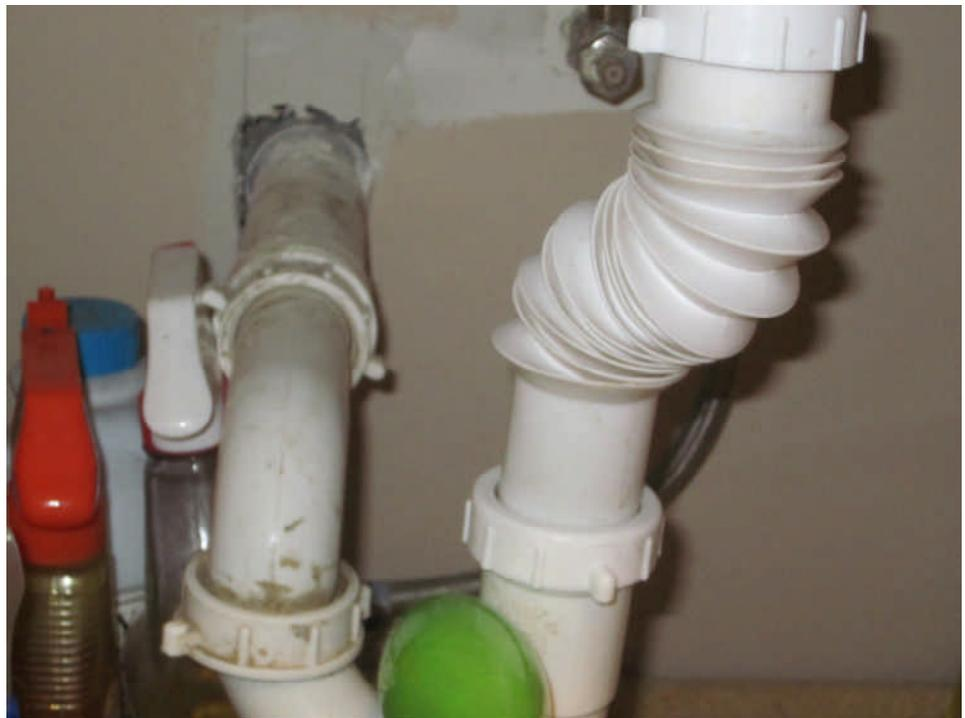
I recommend replacing the flexible plastic drain line under the basement kitchen sink.
