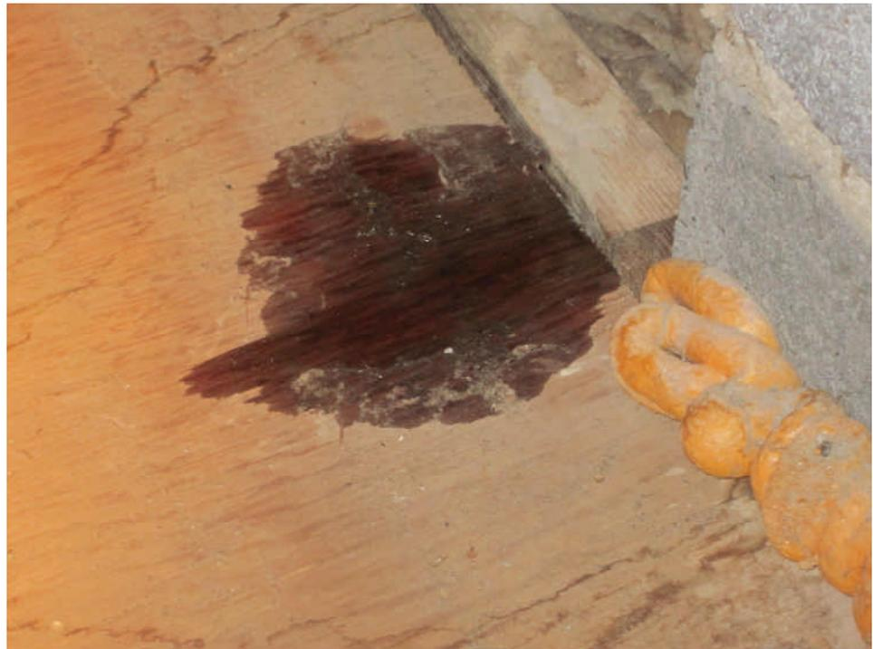
**Action Necessary** - There is evidence of a current leak noted on the underside of the roof decking or rafters.
