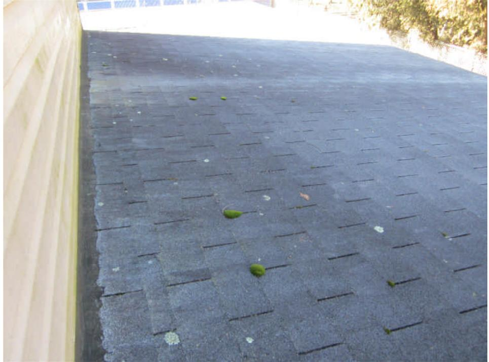
**Attention Needed** - The roof covering material shows signs of deterioration or damage that needs attention to prevent further deterioration or leakage. Moss build up is noted on the right side roof and lose of granulars is noted on the rear lower area roof.
