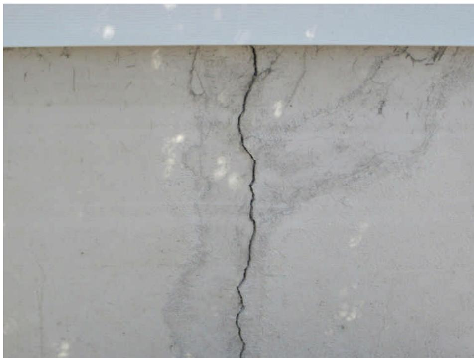
Vertical cracks were noted in the left side exterior wall. Repairs have been made in the past. This home has been flooded in the past.
